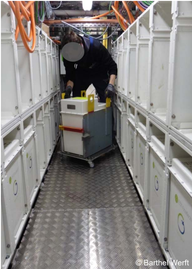
Fitting of accu racks
